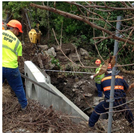
DPW crews install a drainage structure
